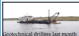
Geotechnical drilling last month
