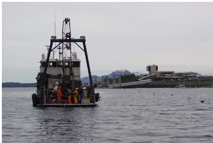
Drilling in Tongass Narrows explored subsurface conditions
